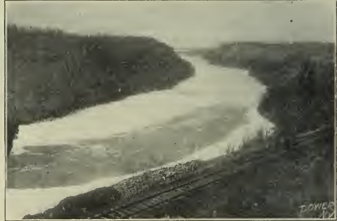
FIG. 2. THE TRACKS OF THE GORGE ROAD ARE BURIED UNDER THE ICE ALL ALONG THE SHORE TO THE RIGHT
